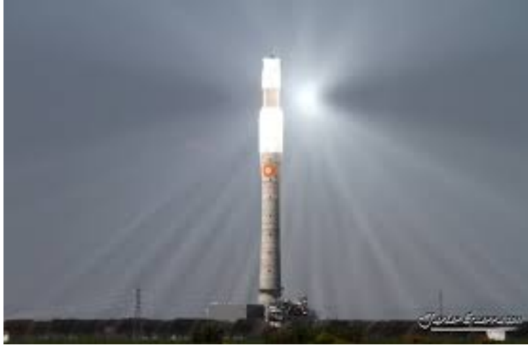
Figure 3 . Radiative losses due to extinction in a solar tower plant.
