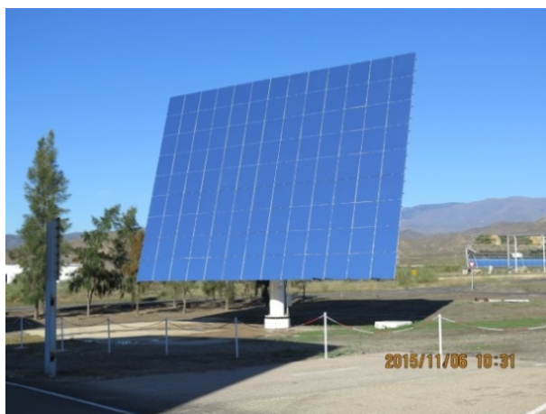
Figure 24. HT120 heliostat with new PSA facets.
