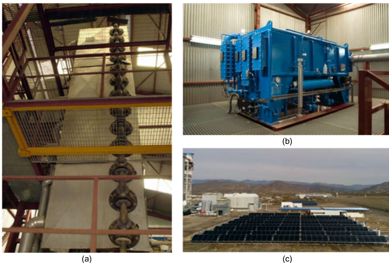
Figure 31. The PSA SOL-14 MED Plant (a) double-effect LiBr-H 2 O absorption heat pump (b) and 606-m 2 flat plate solar collector field (c).
