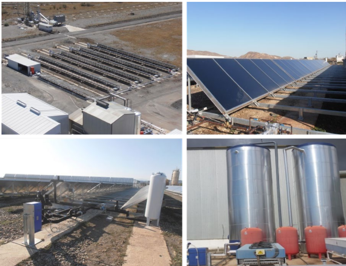
Figure 32. The 606-m 2 large-aperture flat plate solar collector field (AQUASOL-II).
