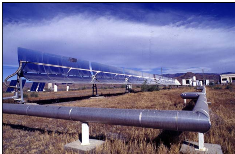
Figure 1. Medium concentration solar collector. One-axis parabolic trough collector (PSA, Spain)
