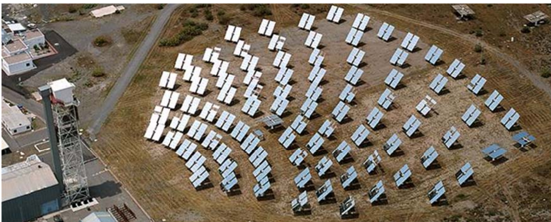
Figure 7. Aerial view of the experimental SSPS-CRS facility.
