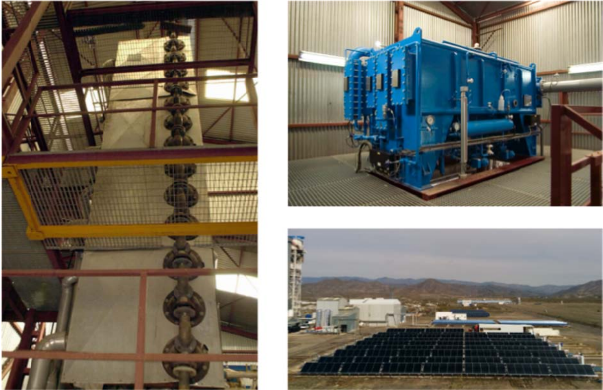
Figure 29. The PSA SOL-14 MED Plant (left), double-effect LiBr-H 2 O absorption heat pump (upper right) and 606-m 2 flat plate solar collector field (bottom right)
