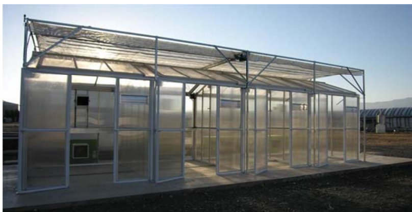
Figure 68. Cultivation chamber for wastewater crops irrigation reuse at PSA facilities.
