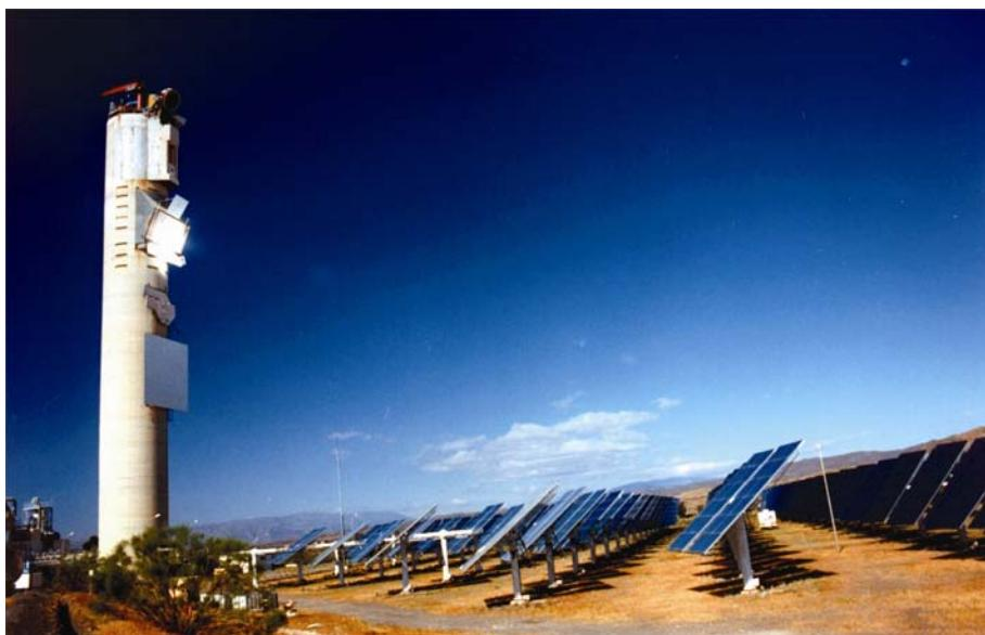
Figure 2.2 The CESA-I facility seen from the East with heliostat rows focusing on the medium-height test level (60 m.)
