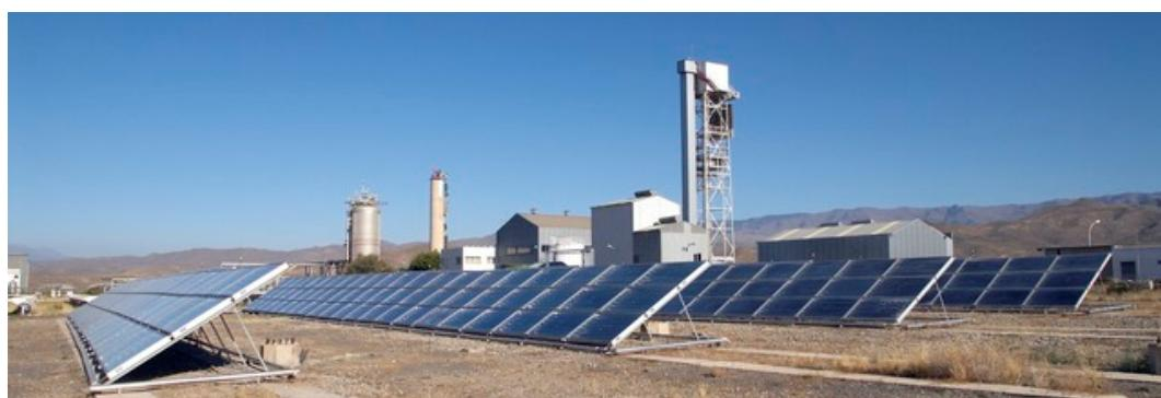
Figure 2.14 SOL-14 plant stationary solar collector field (500 m<sup>2</sup>)
