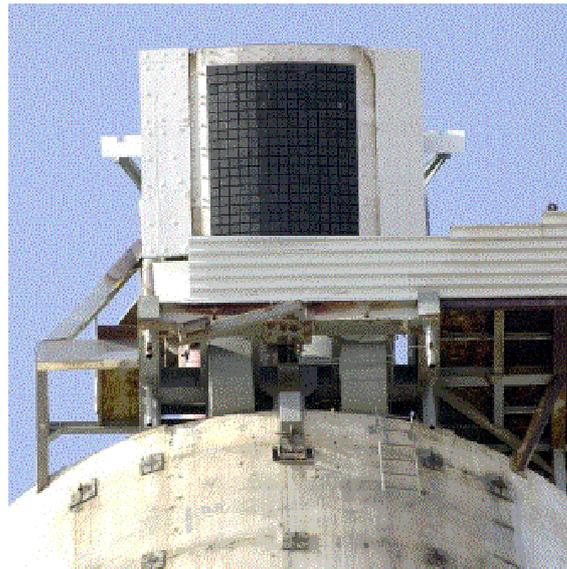
**Figure 40.** The metal absorber TSA receiver being lowered from the tower in March 2003 (left) and front view of the new Solair-3000 receiver in the CESA-I tower.
