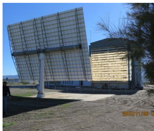
Figure 28. Shutter of the PSA SF-60 Solar Furnace.
