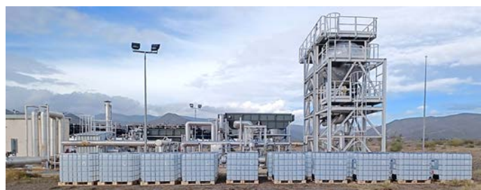
Figure 95. View from the South of the balance of plant of the PTTL test facility, with the IBCs of the new Si-HTF to be tested ready on-site.
