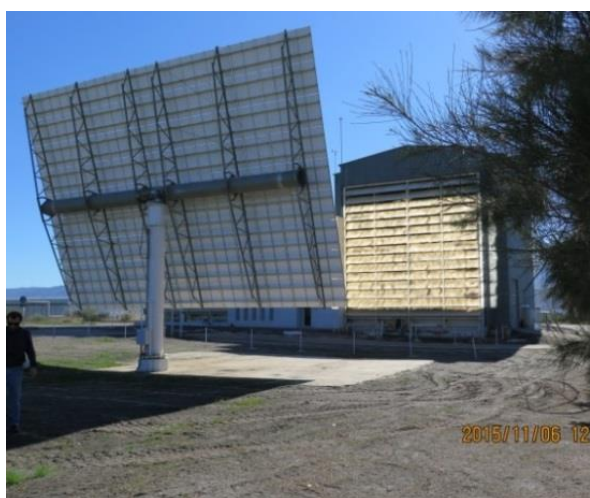
Figure 27. Shutter of the PSA SF-60 Solar Furnace.
