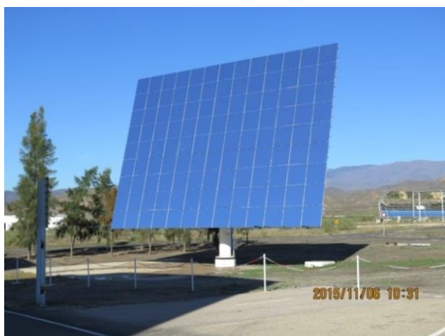
Figure 25. HT120 heliostat in tracking.
