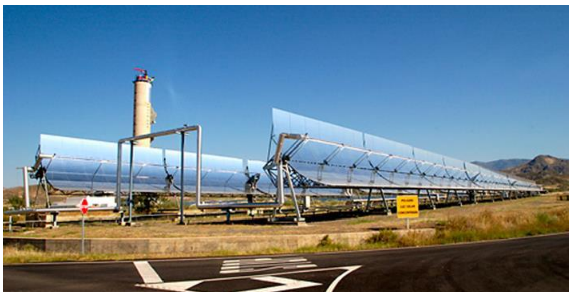
Figure 7. View of the DISS plant solar field in operation.
