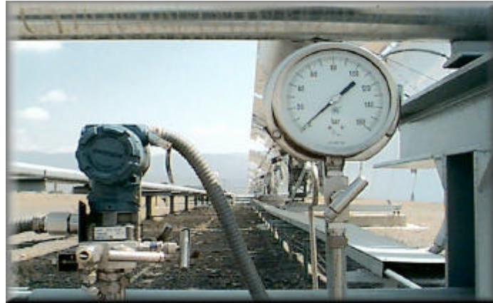
Fig. 3.12 DISS instruments assembly
