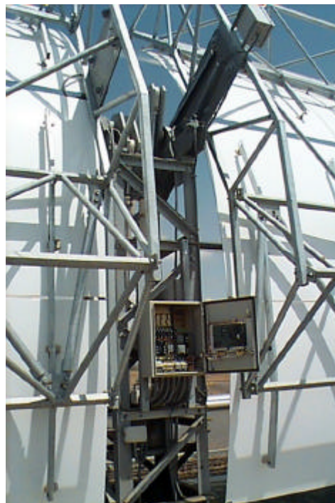
Fig. 3.13 DISS Local Controller assembly
