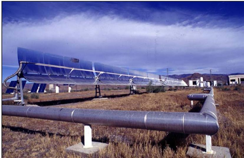
**Figure 4.1.** Medium concentration solar collector. One-axis parabolic trough collector (PSA, Spain)
