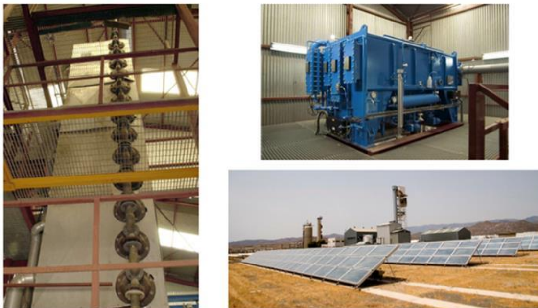
Figure 2.31. The PSA SOL-14 MED Plant (left), double-effect LiBr-H 2 O absorption heat pump (upper right) and 500\text{-m}^2 CPC solar collector field (bottom right)
