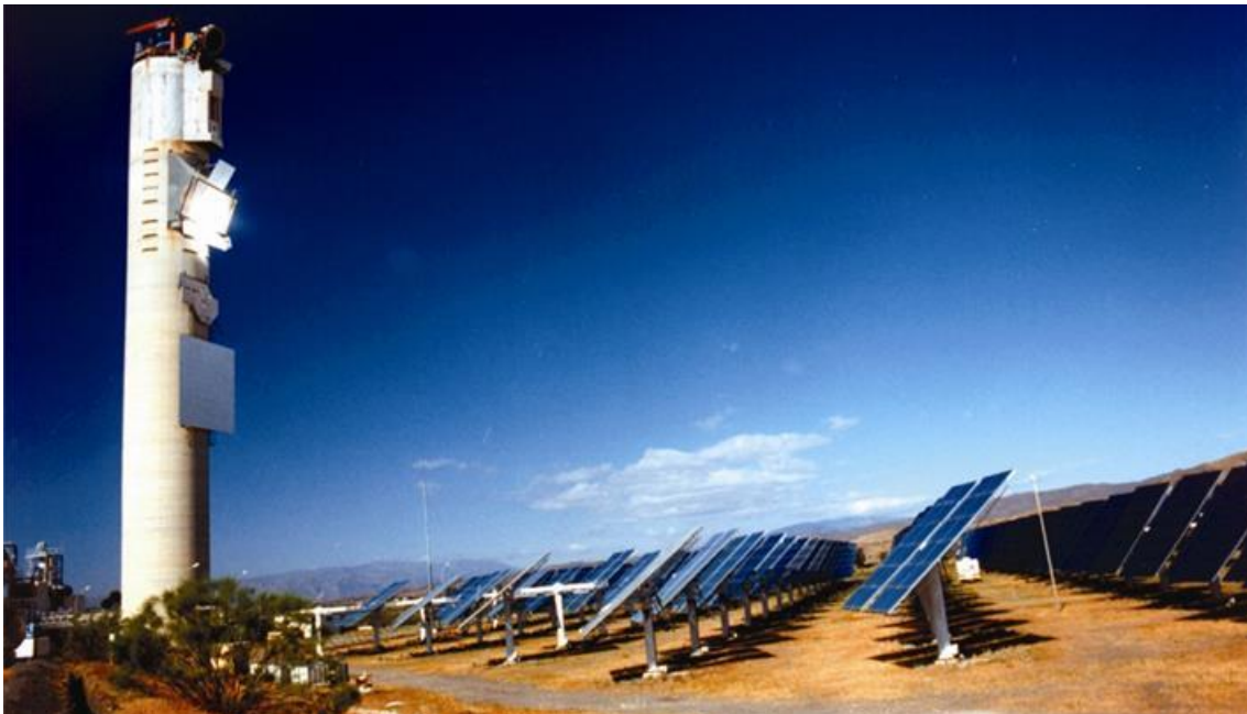
Figure 2.2. The CESA-1 facility seen from the East with heliostat rows focusing on the medium-height test level (60 m)
