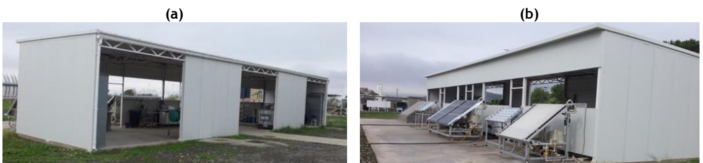
Figure 2.38. North (a) and south (b) view of the new hangar to accommodate new installations.
