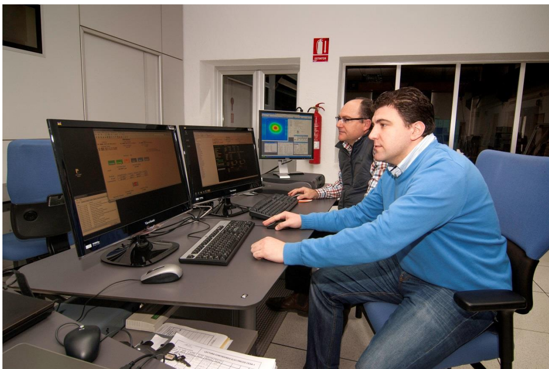
Figure 3.14. Central control room of the heliostat field.
