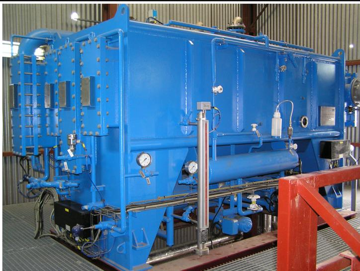
Figure 4.31. Double-effect absorption heat pump (LiBr-H<sub>2</sub>O) at the PSA
