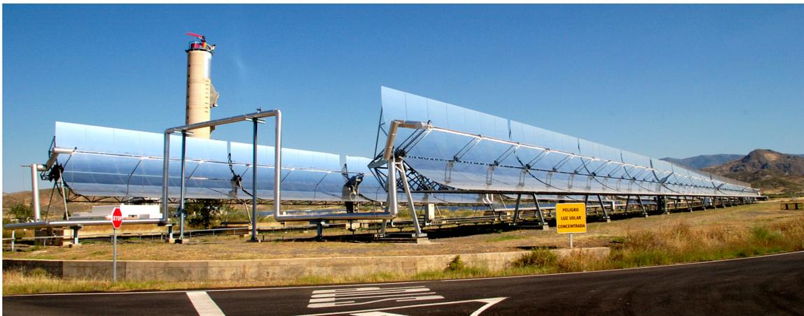
Figure 2.7. View of the DISS plant solar field in operation
