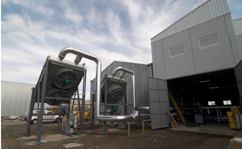
Figure 2.52. View of the outside of the CSP+D test bed building and the air coolers that act as the condensers in a conventional power cycle configuration.
