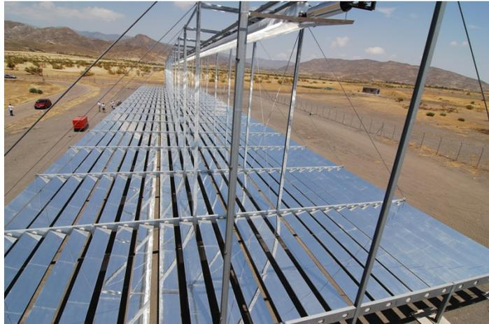
Figure 2.10. Photo of the MAN linear Fresnel demo collector erected on the Plataforma Solar de Almería (PSA).
