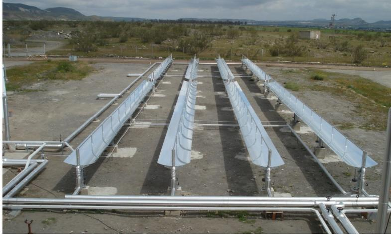
Figure 2.55. NEP-Polytrough 1200 solar field
