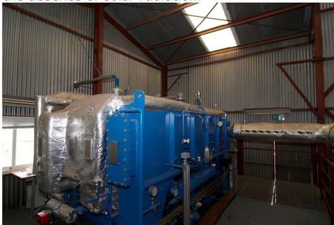
Figure 2.45. Double effect BrLi-H<sub>2</sub>O absorption pump hooked up to the MED plant
