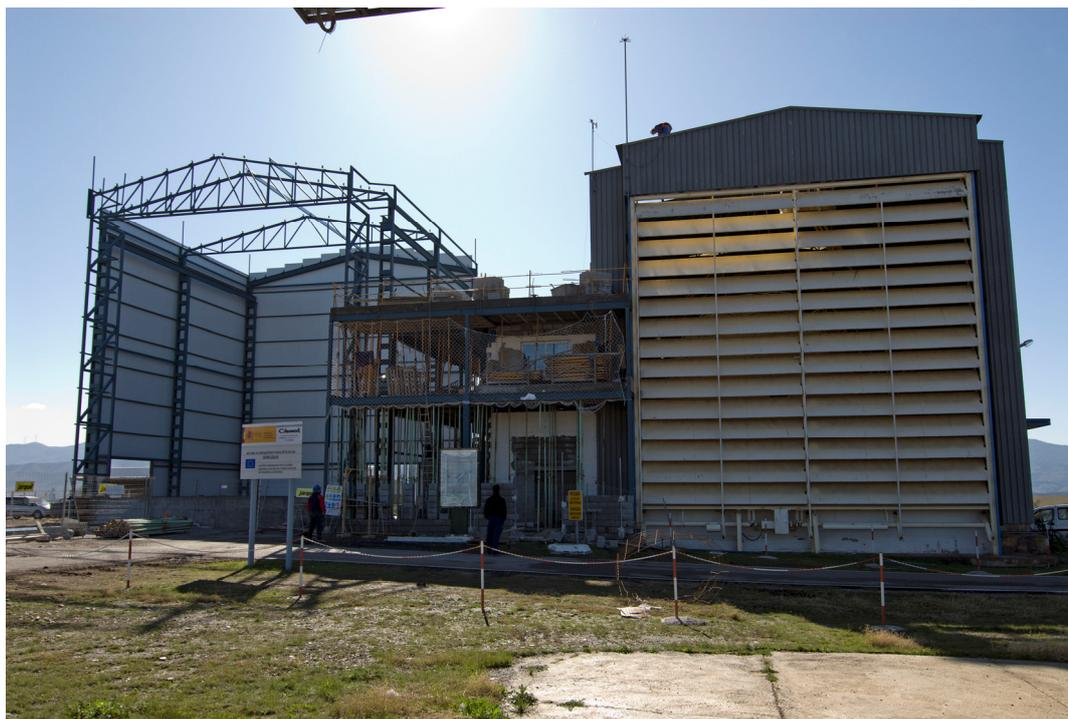
Figure 2.40. The new solar furnace under construction
