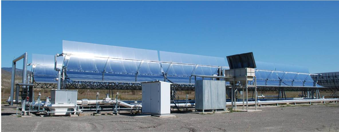
Figure 3.9 View of the experimental loop used in 2008 and 2009 to study pressurized gas in parabolic trough collectors
