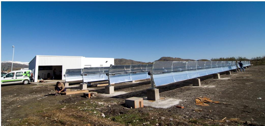
Figure 2.41. New collectors for generating saturated steam
