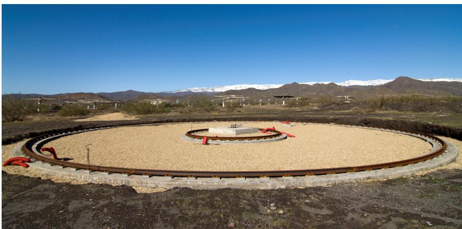
Figure 2.39. Foundations of the new 'Kontas' installation for characterization of PTCs
