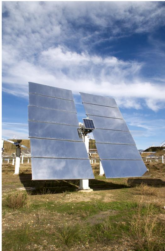
Figure 2.3. An autonomous heliostat in the CRS field
