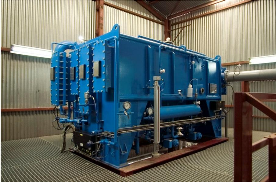
Figure 4.14 Double effect (LiBr-H<sub>2</sub>O) absorption heat pump
