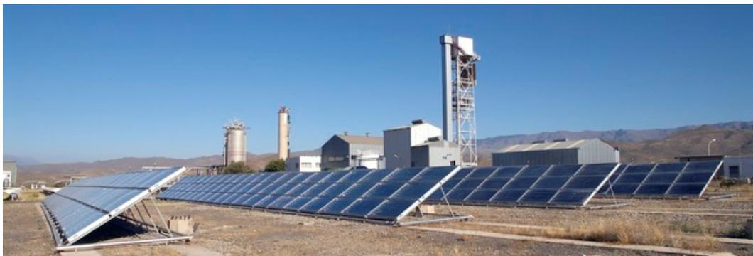
Figure 2.14 SOL-14 plant stationary solar collector field (500 m<sup>2</sup>)
