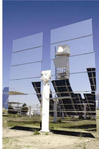
Figure 2.3 A CRS field heliostat reflecting the tower
