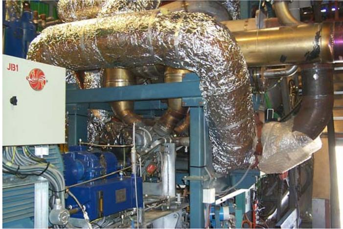
Figure 3.17 Ormat turbine at the 60-m level in the CESA-1 tower
