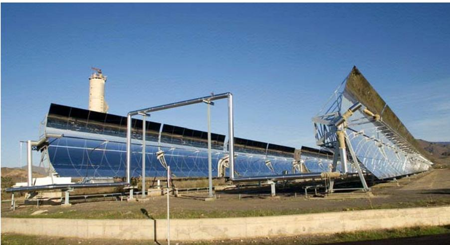
Figure 50. View of the "U-shape" connection between the two new collectors and the row installed in 1998.
