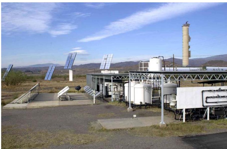
**Figure 25. General view of the CPC Solar Photochemical Facilities with the new collector in the foreground**
