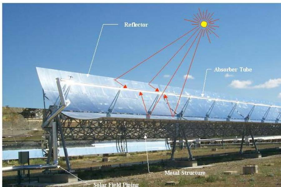
**Figure 46. The parabolic-trough collector principle**
