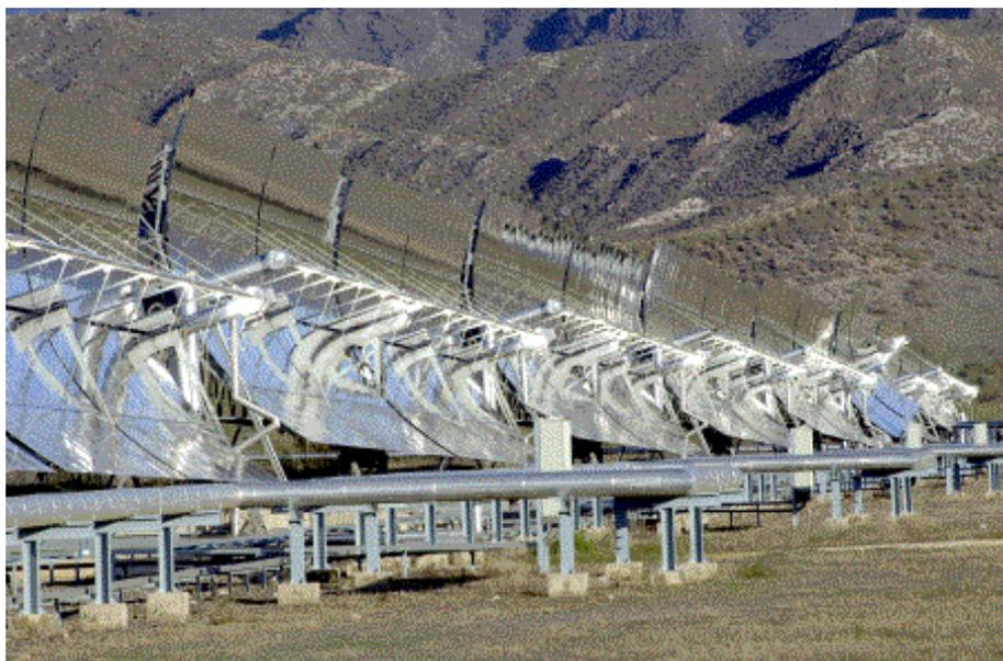
Figure 10. View of the DISS plant solar field in operation
