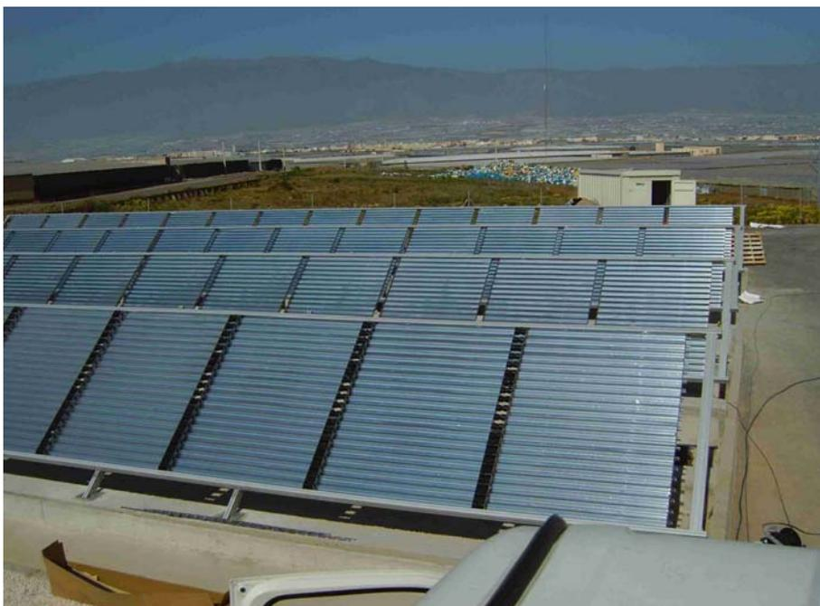
Figure 60. Partial view of the plant solar collector field during erection
