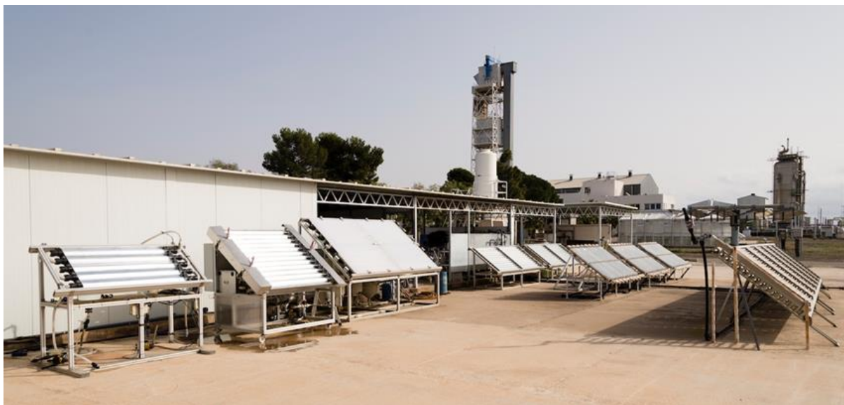
Figure 35. View of several CPC photo-reactors for purification of water.
