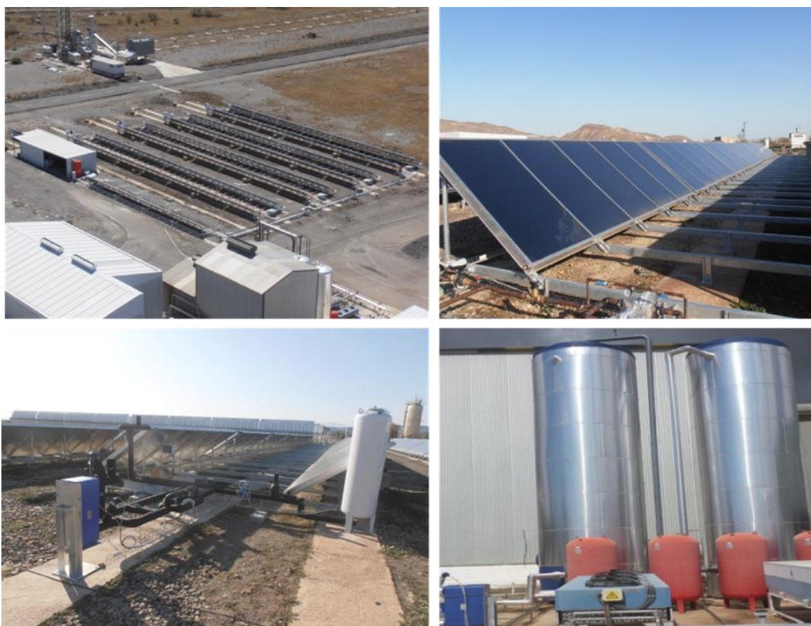
Figure 28. The 606-m 2 large-aperture flat plate solar collector field (AQUASOL-II).
