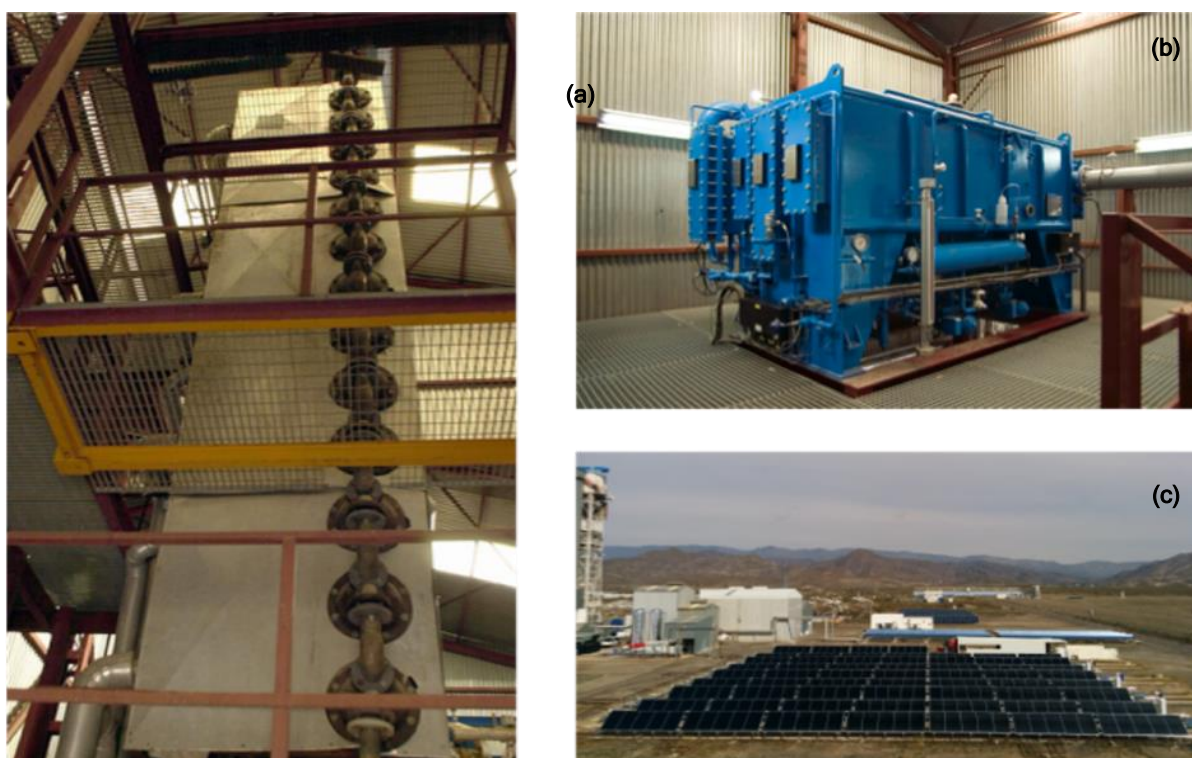
Figure 27. The PSA SOL-14 MED Plant (a), double-effect LiBr-H 2 O absorption heat pump (b) and 606-m 2 flat plate solar collector field (c).
